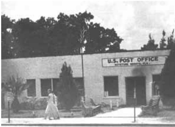
Hazel McKay can be seen strolling by former Post Office.
